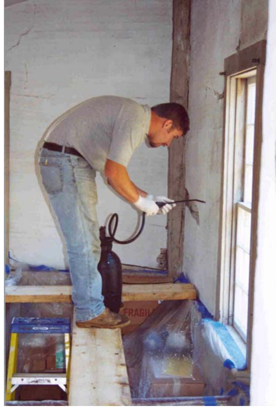
Figure 13 & 14. Joe Serra cleaning and pre-wetting areas of damaged plaster prior to consolidation.
