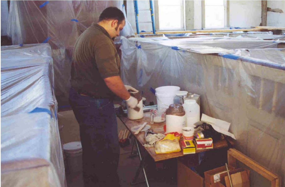
Figure 12. Joaquim da Fonseca preparing plaster consolidant materials.
