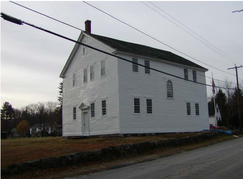
Figure 23. View from northeast.
