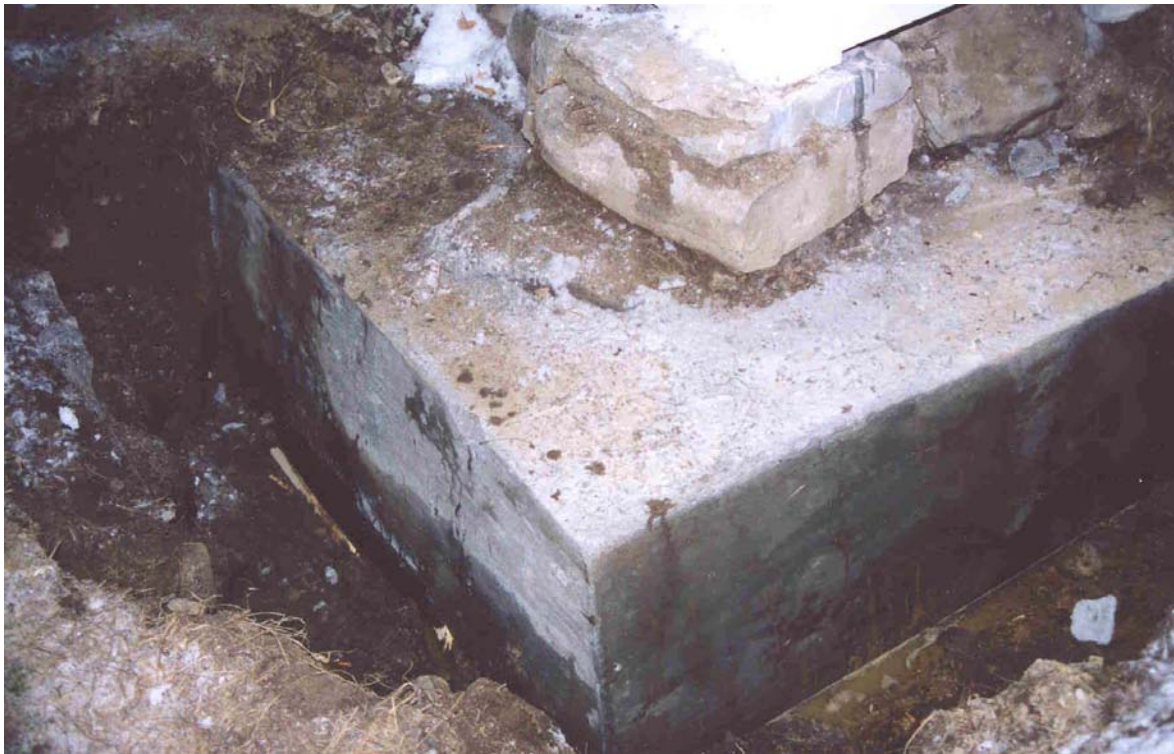
Figure 7. Finished concrete footing in place at northwest corner of building.
