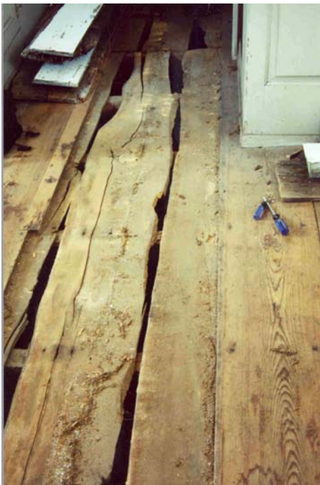
Figure 10 & 11. Before and after photographs showing subfloor and finished floor reinstated after borate treatment.
