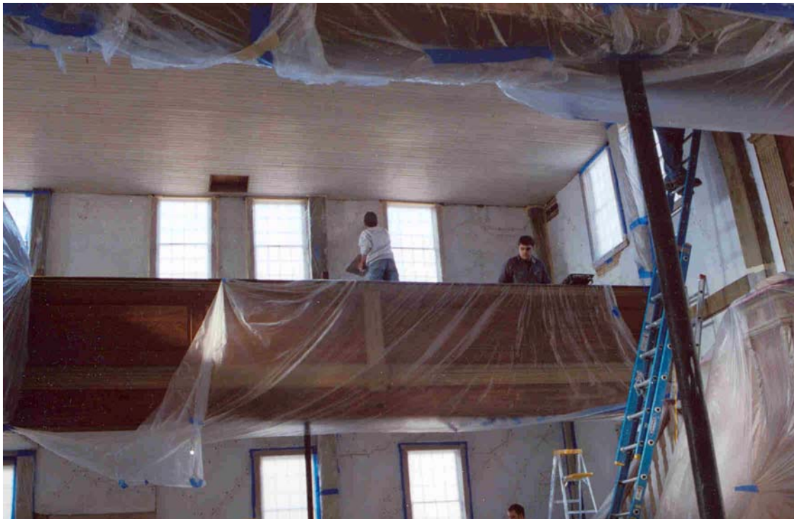
Figure 15. Plaster repairs following consolidation.
