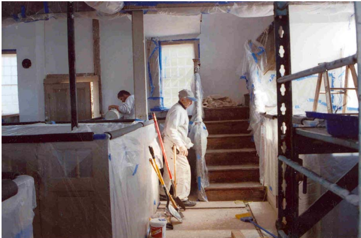
Figure 17. Plasterer Frank. J. Mangione of Saugerties, NY completing interior plaster repair.
