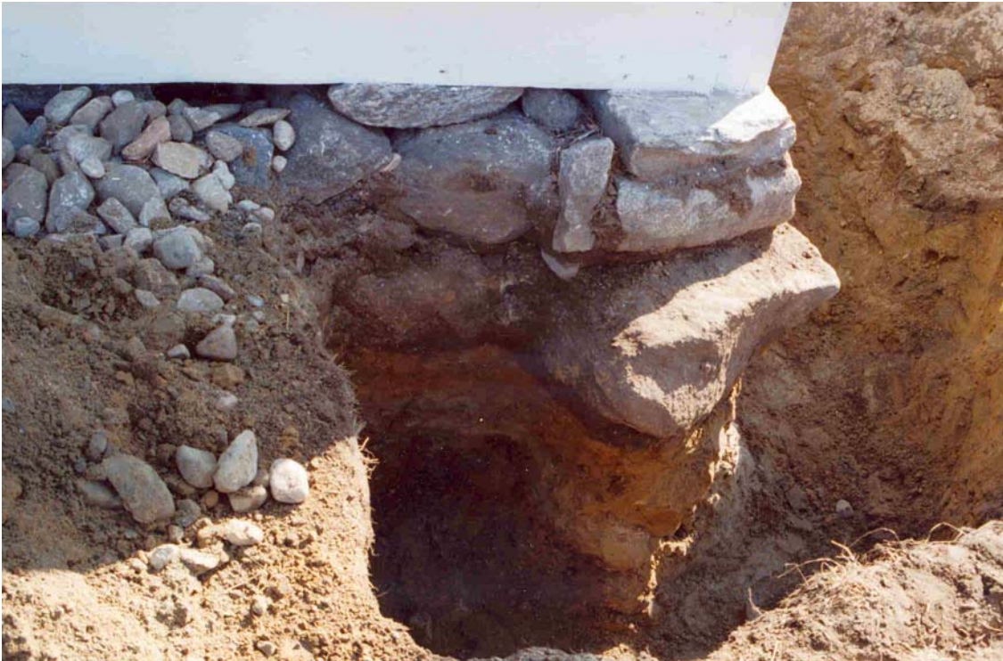
Figure 5. Northwest corner of building excavated to show original stone footing.
