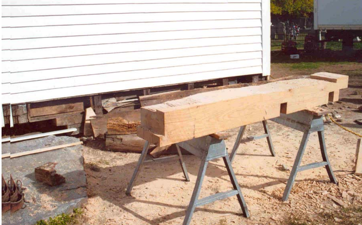
Figure 3. New section of White Oak sill fabricated and ready for installation.
