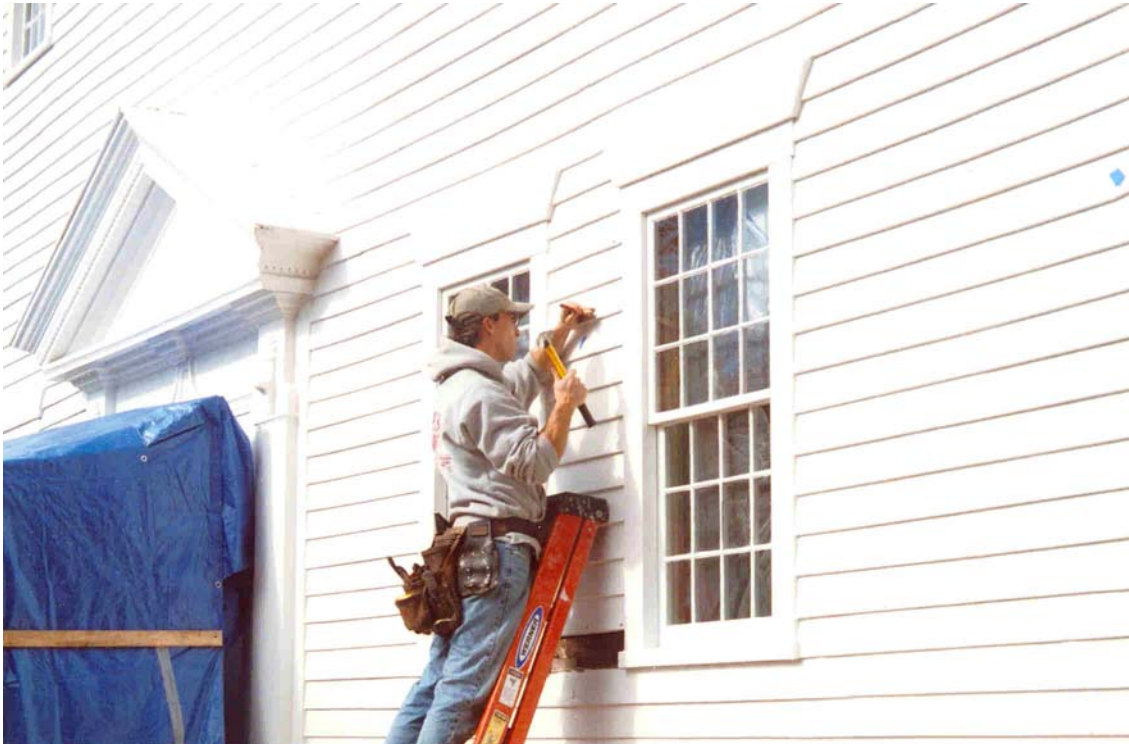
Figure 20. Exterior millwork replair
