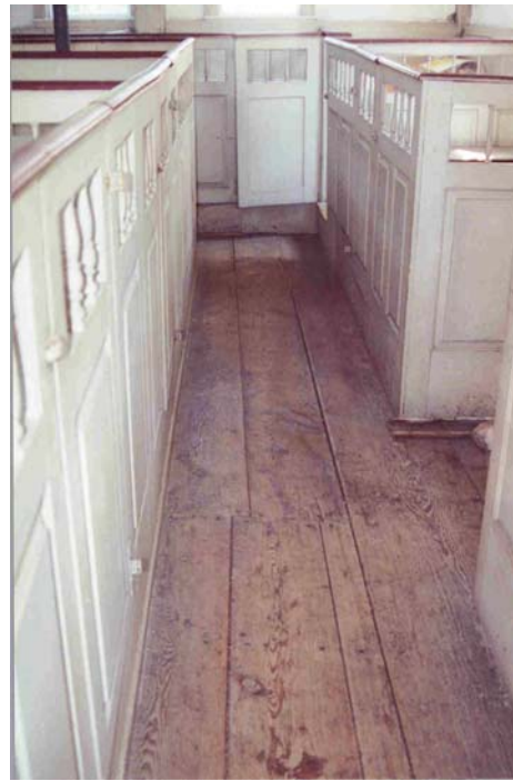
Figure 10 & 11. Before and after photographs showing subfloor and finished floor reinstated after borate treatment.
