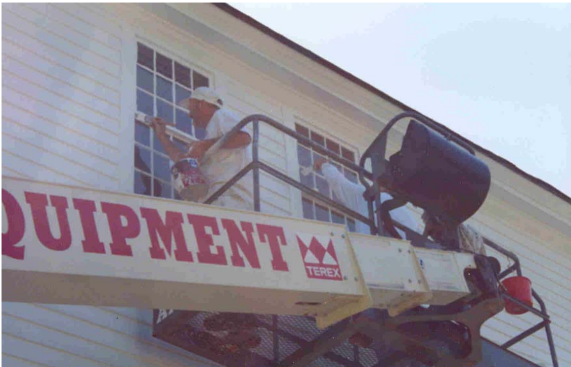
Figure 21. Exterior painting using bucket truck.
