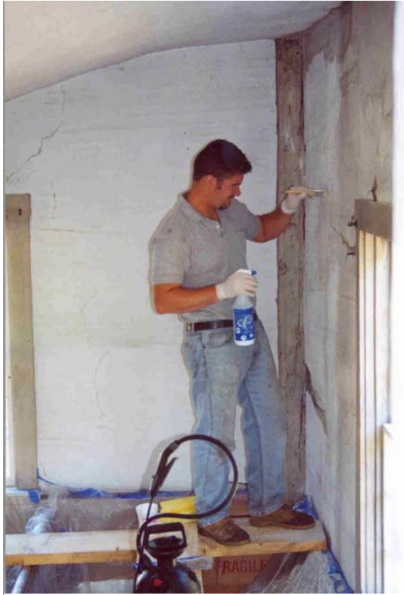
Figure 13 & 14. Joe Serra cleaning and pre-wetting areas of damaged plaster prior to consolidation.
