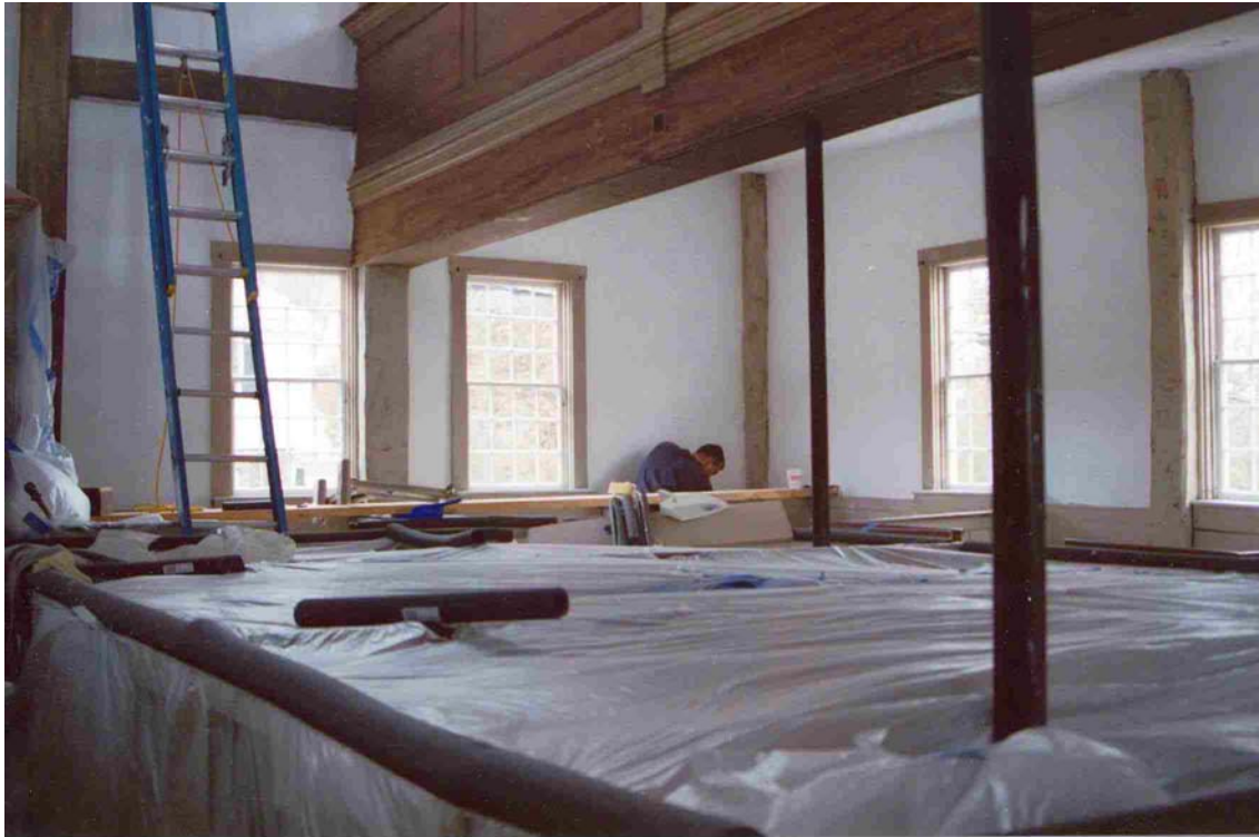
Figure 18. Completing interior whitewashing.
